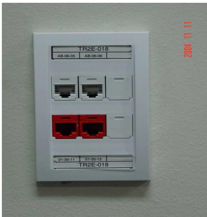
Figure 2 – Wall Area Outlet Faceplate Labeling.
