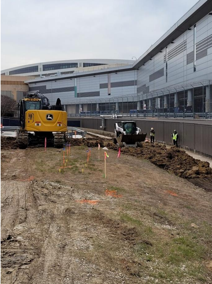
Demolition at future South Pump Room Area
