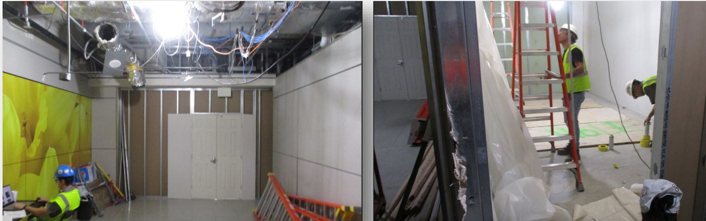
A12 SSCP Construction Progress – Aug 5
