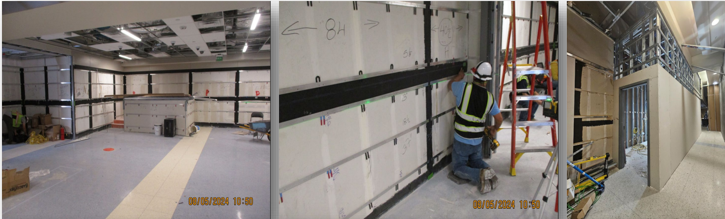
A21 SSCP Construction Progress – Aug 5
